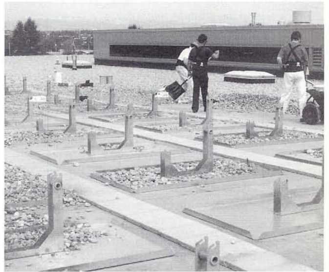
Above: Gravel holds roof jacks to roof.
